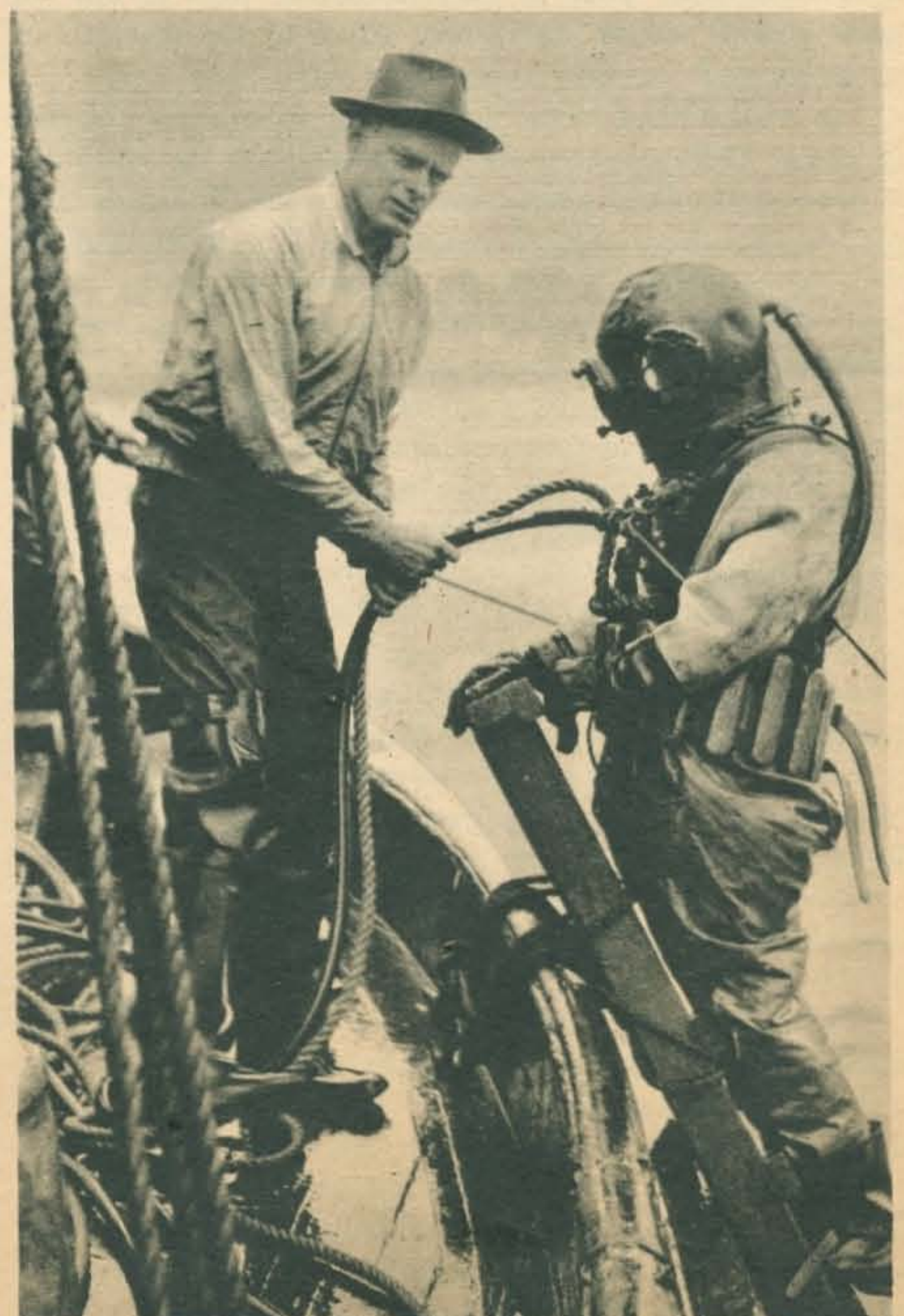
DIVERS LAY POWER AND COMMUNICATION LINES TO THE MAINLAND
